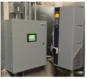
AirTest CN7232 Garage Controller with Danfoss VFD installed in St Francis Hotel at Union Square in San Francisco.
